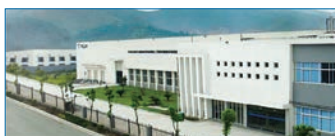
Suzhou, China Velan Valve (Suzhou) Co. Ltd.
