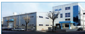
Plant 1: Ansan City, South Korea Velan Ltd.
