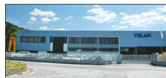
Lucca, Italy Velan ABV S.r.l., Plant 1
