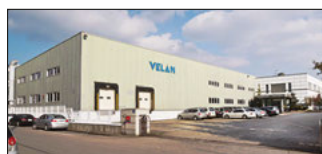
Ansan City, South Korea Velan Ltd., Plant 2
