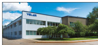
Williston, VT, U.S.A. Velan Valve Corp., Plant 3
