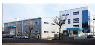
Ansan City, South Korea Velan Ltd., Plant 1
