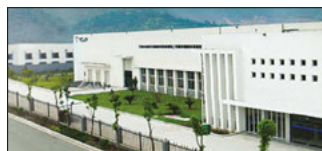
Suzhou, China Velan Valve (Suzhou) Co., Ltd.
