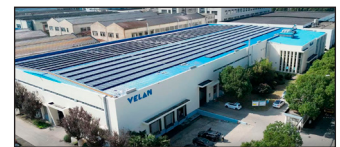
Suzhou, China Velan Valve (Suzhou) Co., Ltd.
