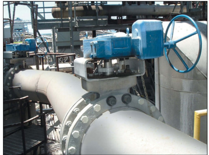
Torqseal™ triple-offset valve application.
