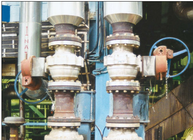
Two 8" (200 mm) Velan Securaseal® metal-seated liquor isolation valves.
