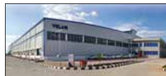
Coimbatore, Inde Velan Valves India Pvt. Ltd.
