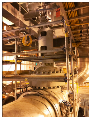
Gasket replacement on a 30" Velan bolted bonnet gate valve
