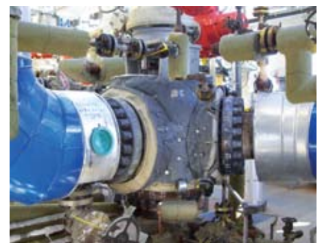
A Velan coker switch valve in service in a European refinery. Velan is a leading supplier of coker ball valves worldwide.
