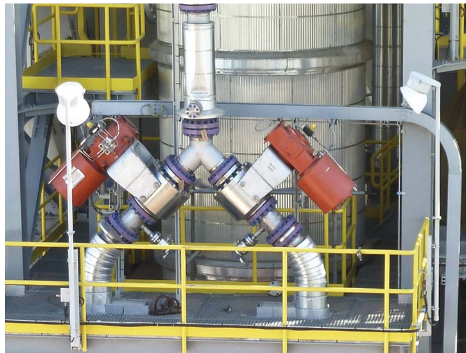
Two 10" Class 150, super duplex, stainless steel Velan Securaseal valves.
